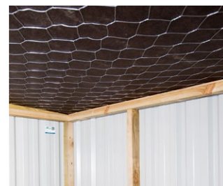
Paper and netting* for extra protection from moisture and condensation.
