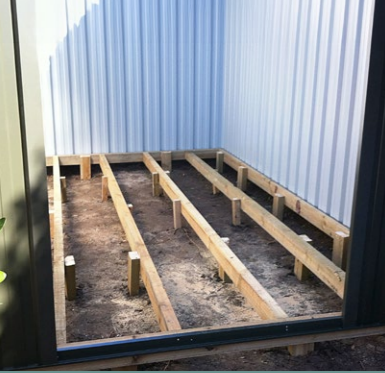
H4 treated timber subfloor
