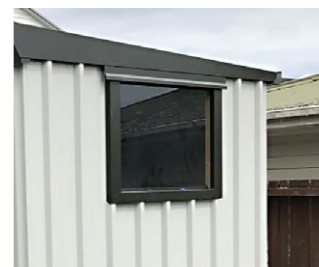
Fixed glass window for added natural light.
